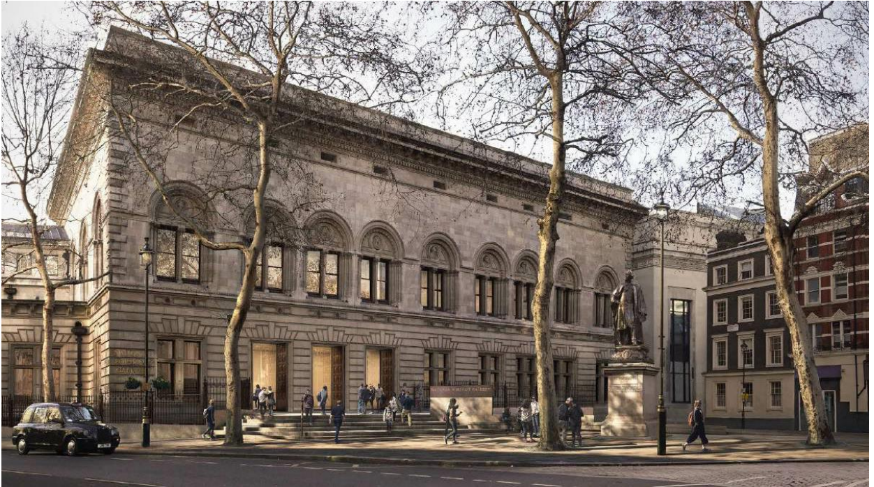
Computer Generated Image of Northern Façade
